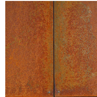
Corten steel retaining wall
