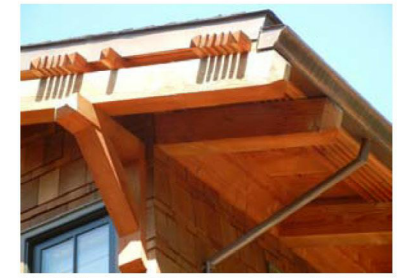
Building with copper flashing, gutter and drainpipe.
