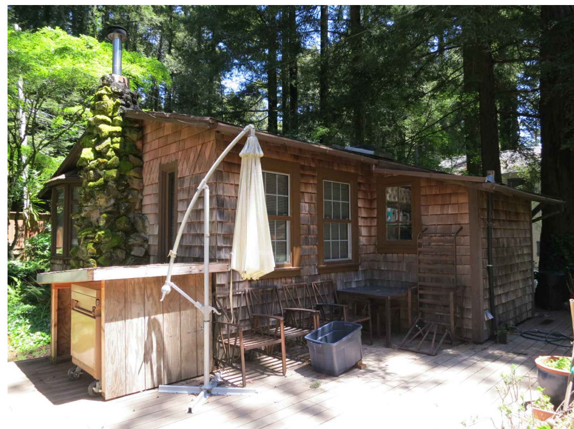
PHOTO F: PARTIAL REAR ELEVATION
