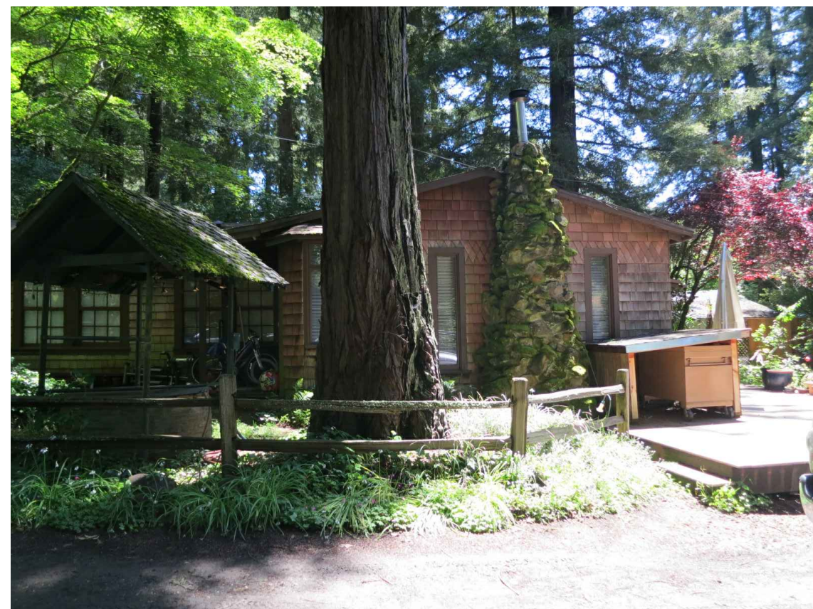
PHOTO D: PARTIAL WEST ELEVATION
