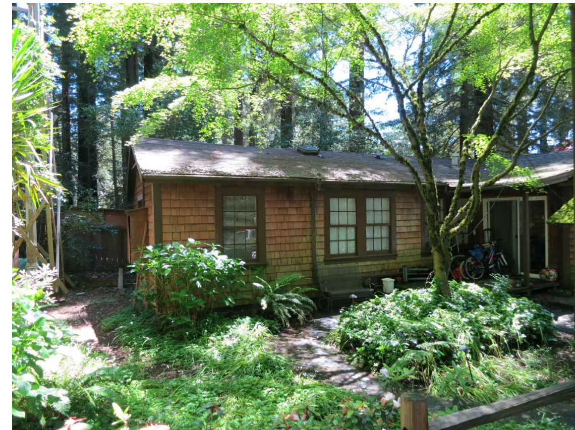
PHOTO A: PARTIAL WEST ELEVATION @ FRONT
