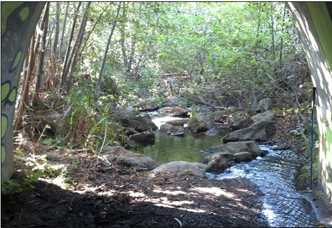
Photograph 8. Looking downstream (southwest) along Whitehouse Creek through culvert beneath SR 1 towards riparian forest west of the project footprint.
