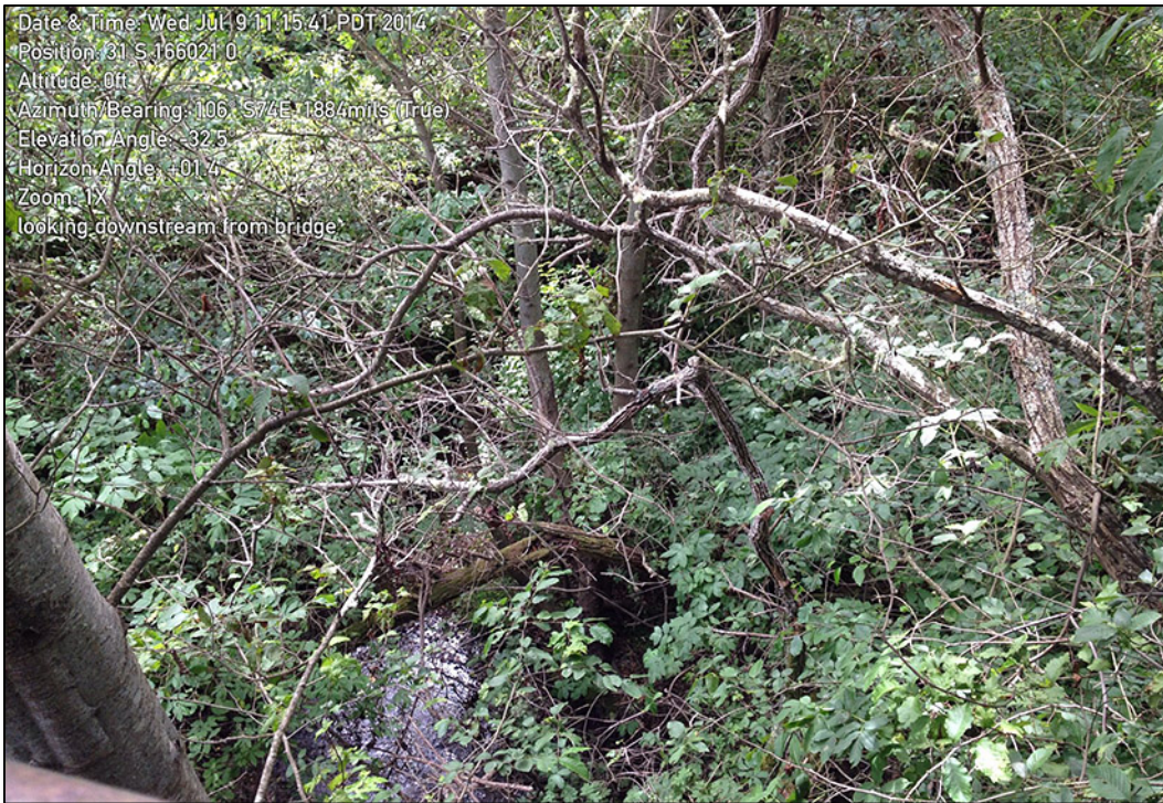
Photograph 4. Whitehouse Creek, looking downstream (south-southeast) from pedestrian bridge along existing trail approximately 800 feet upstream from the biological study area.
