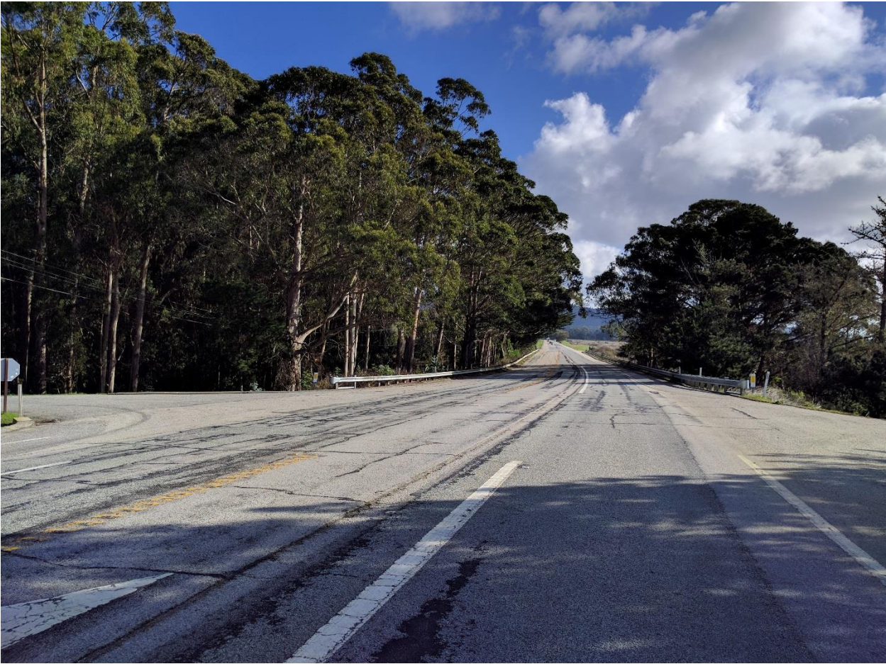
View from Southbound State Route 1
