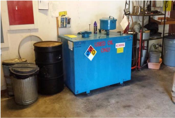
Photo 7: View of waste oil containment inside Apparatus Building.
