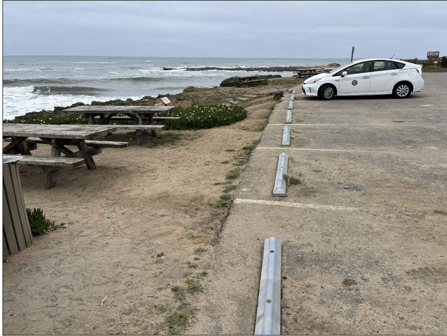
Photograph 15. View looking west towards an accessible picnic table location at the Bean Hollow State Beach Project Area.
