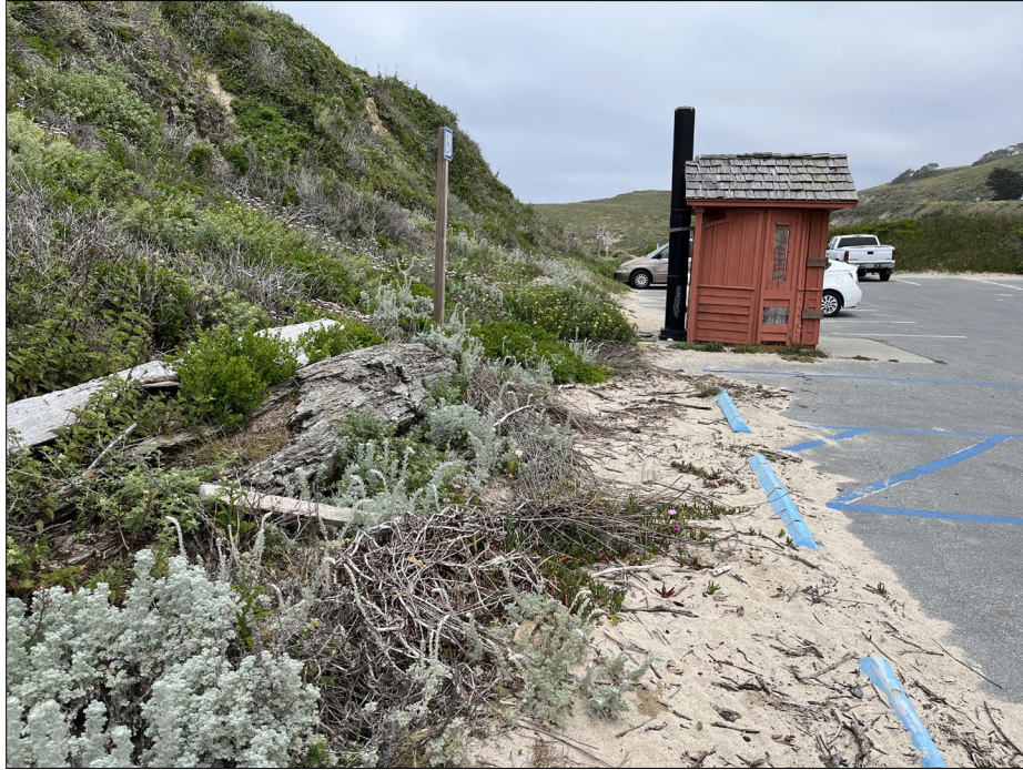
Photograph 11. View looking south towards the restroom to be replaced at the Pescadero State Beach North Project Area.
