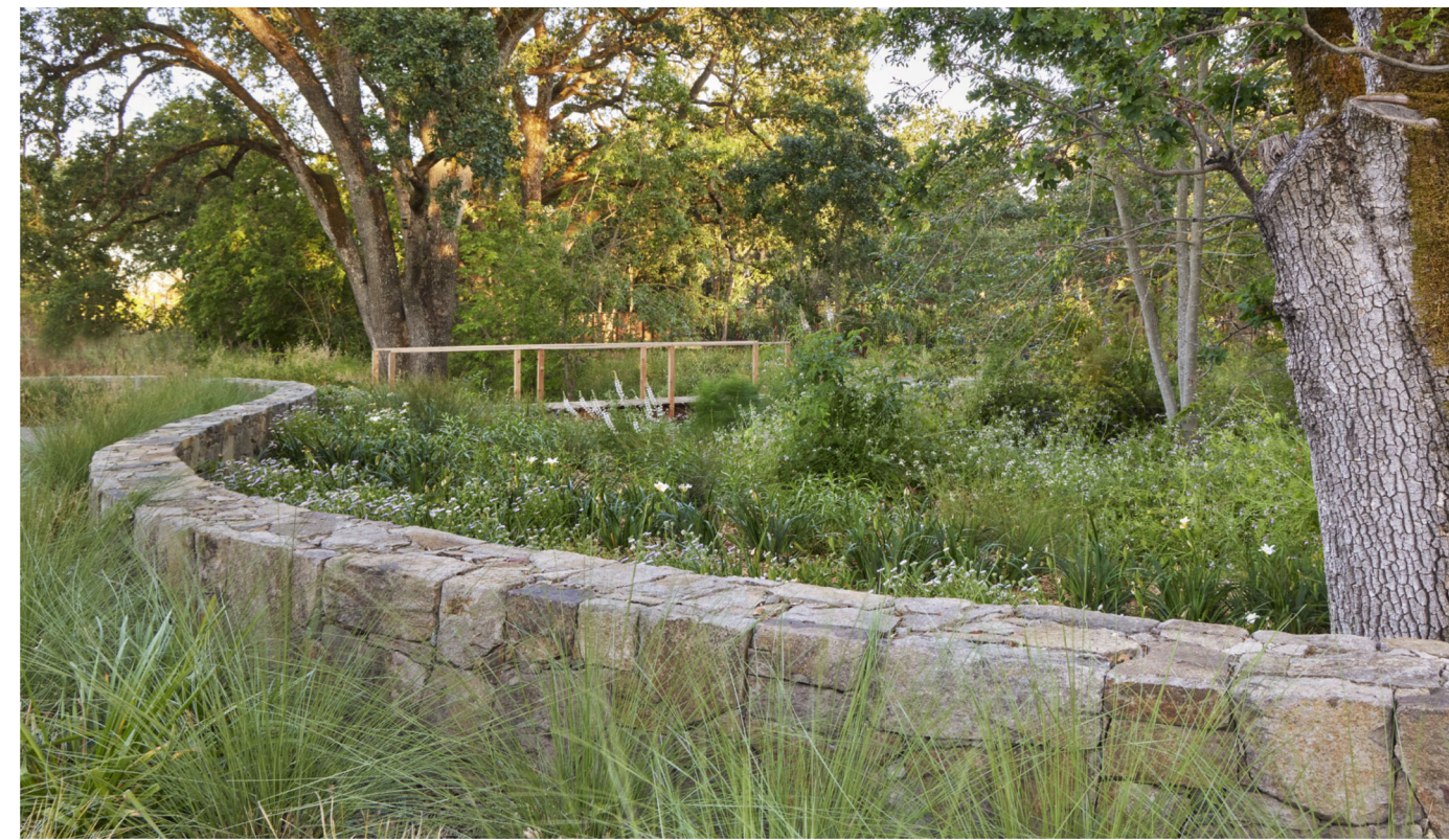
09. STONE RETAINING WALL - EARTH AND GREY TONES. ALL WALLS TO HAVE SAME STONE AND MASONRY TREATMENT
