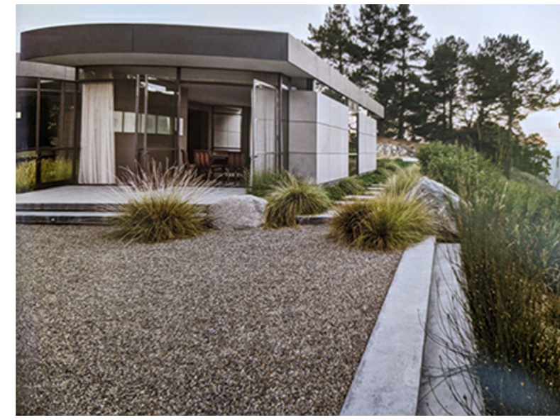
02. GRAVEL PAVING ON CLASS 2 PERMEABLE BASE ROCK AND STABILIZED WITH GEO GRID SUPPLIER: LYNGSO - PRODUCT: 1/8" CALIFORNIA GOLD
