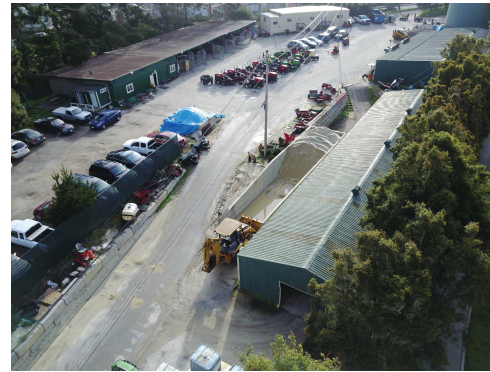
3 VIEW OF SITE LOOKING SOUTH
