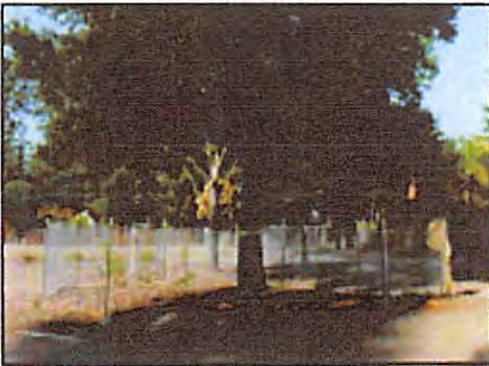
IMAGE 2.15-2 Tree Protection Fence at the Dripline
