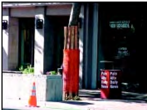
IMAGE 2.15-4 Trunk Wrap Protection
