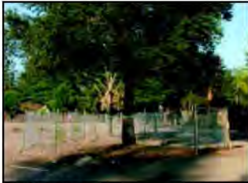
IMAGE 2.15-2 Tree Protection Fence at the Dripline
