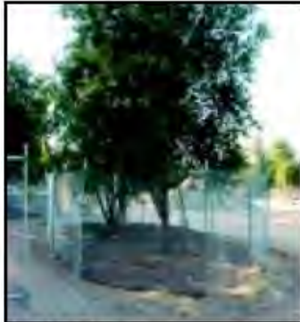
IMAGE 2.15-1 Tree Protection Fence at the Dripline
