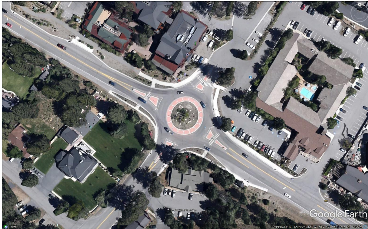
Example of left turn pocket on roundabout departure leg (Martis Valley Drive/Brockway Road Intersection - example from Dan Wilkins)
